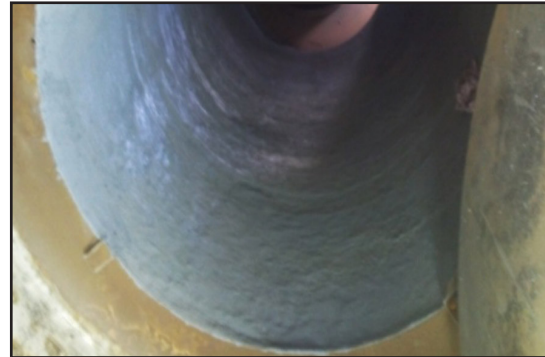
Application of ARC BX1* in one of the cyclones at 6-8 mm
